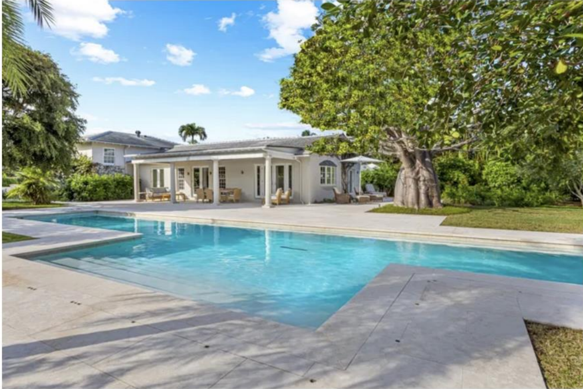
The 1950s-er house that just sold for $14.9 million at 1333 N. Lake Way in Palm Beach has a lap pool built in 2016 on the property's south side. Ryan Walblay, Global Video Pros/Provided By Margit Brandt Of Premier Estate Properties
